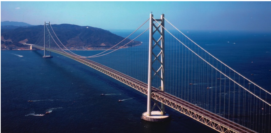
Fig. 5: Suspension Bridge – Akashi Kaikyo Bridge, Japan
