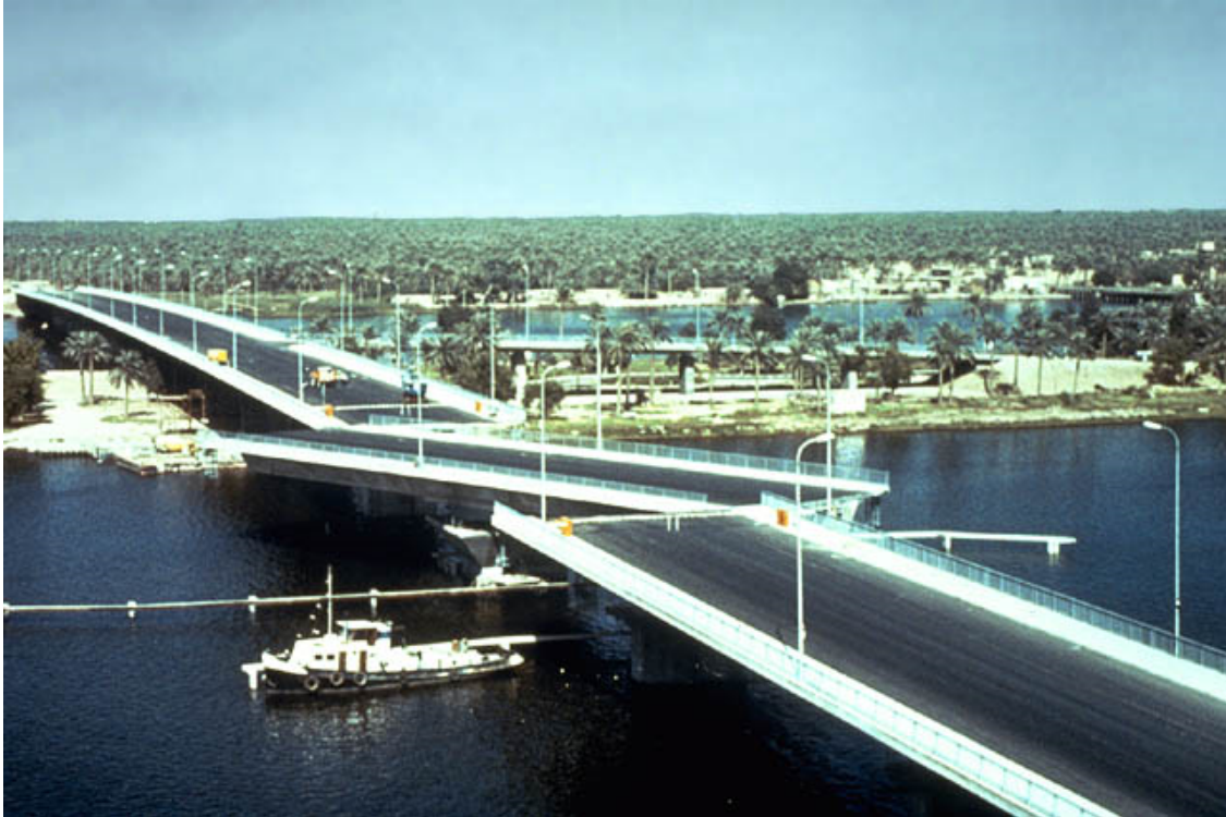
Fig.6: Swing Bridge- ( Bridge Across Shatt-al-arab, Iraq )
