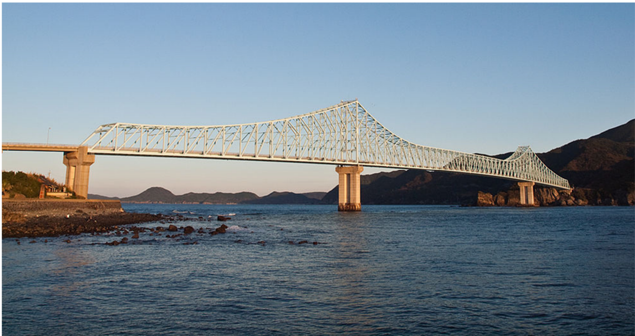
Fig. 3:Truss Bridge – Ikitsuki Bridge, Nagasaki, Japan
