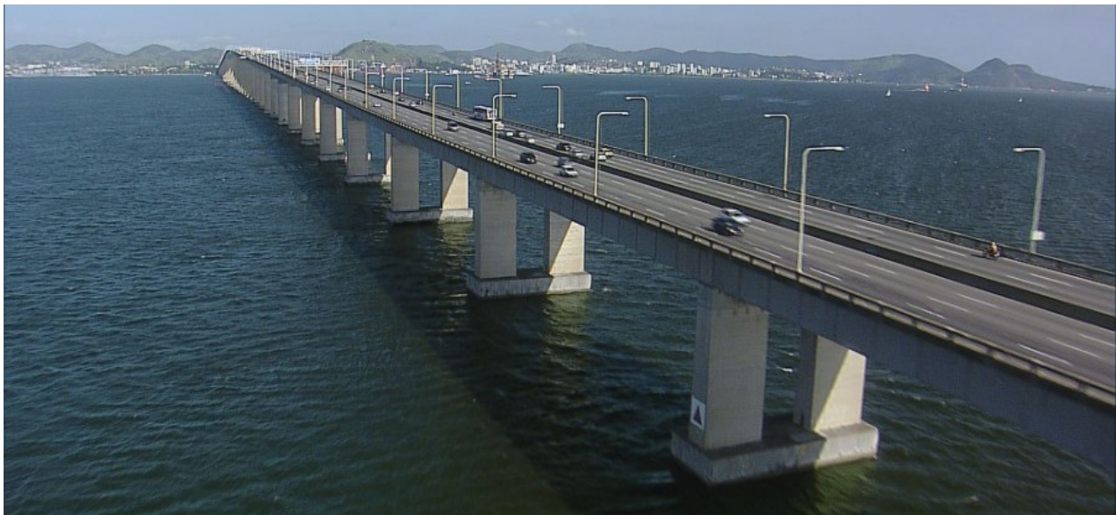
Fig. 1: Deck-girder Bridge – Niteroi Bridge, Rio De Janeiro, Brazil
