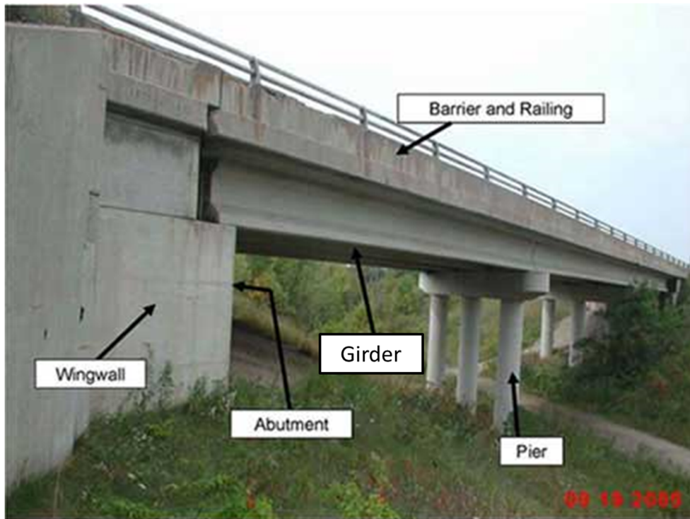
Fig. 8: Different components of a Bridge
