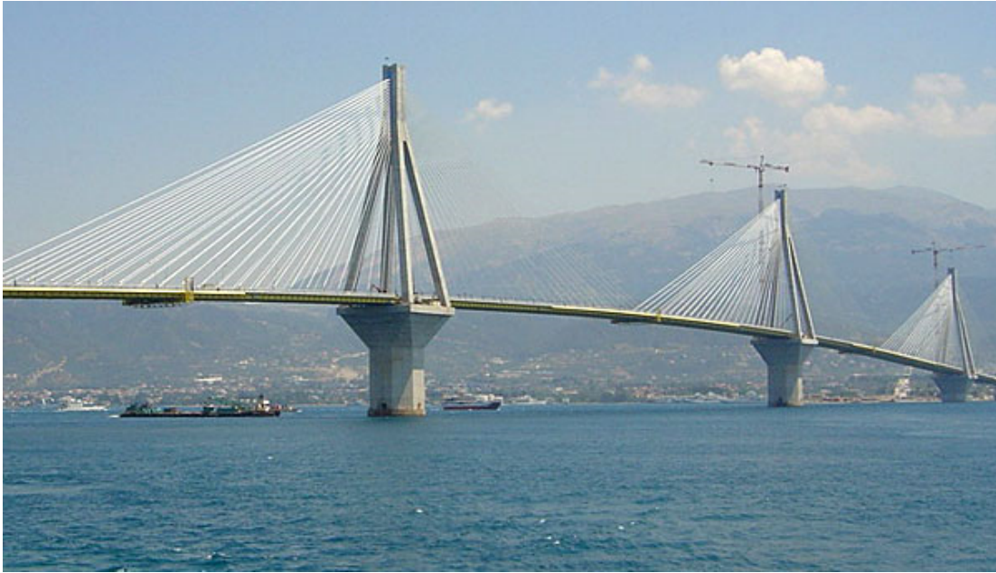
Fig.4: Cable-stayed Bridge – Rion Antirion Bridge, Greece
